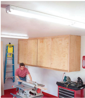
8' Fluorescent With four 4 ft. lamps
